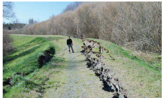
Slumping and lateral spreading observed on stopbanks on Waimakariri River following earthquakes in Sept 2010, Source: Environment Canterbury
